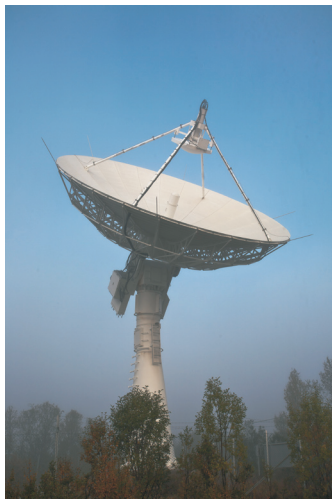
One of the antennas at the antenna area. Photo: KSAT
